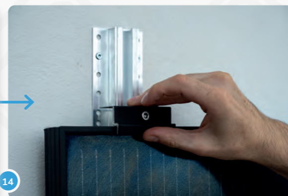
14 Schiene in Position bringen...
